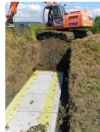
Protections de pipelines
